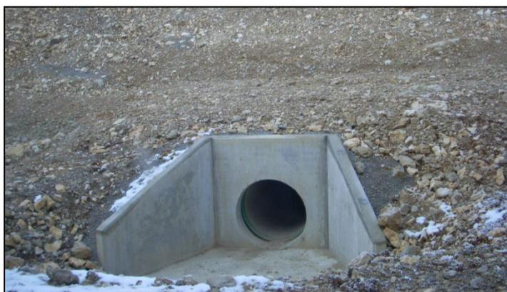
All the various headwalls shall include a cast in-situ cut-off wall, compulsorily poured in situ and in contact with natural ground. This shall be cast in-situ without formwork. This restriction applies also to prefabricated headwalls.
